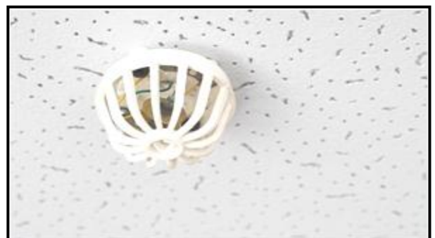
Smoke detectors alert people of the presence of fire.
